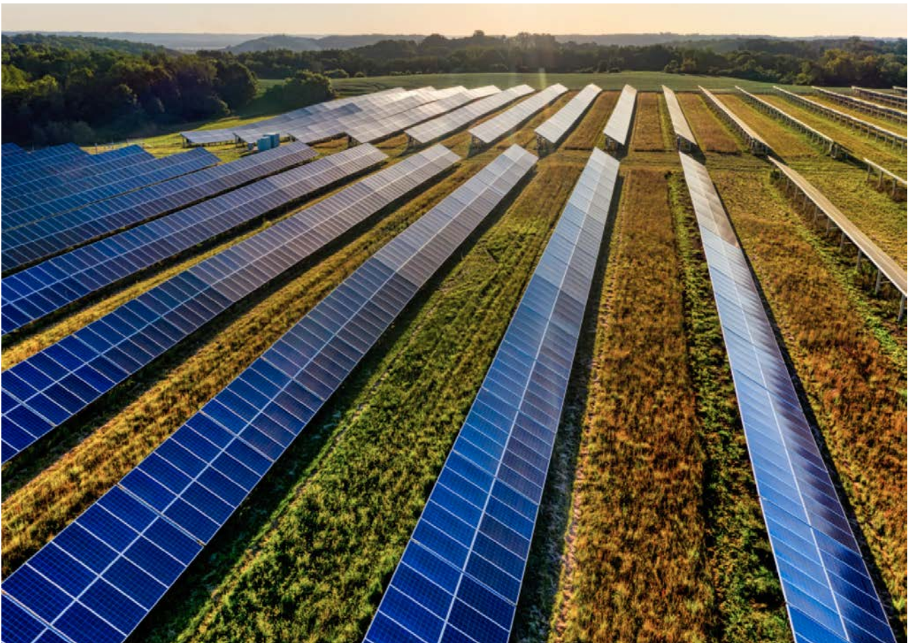
Figure 3. Agrisolar (Source: National Center for Appropriate Technology)
